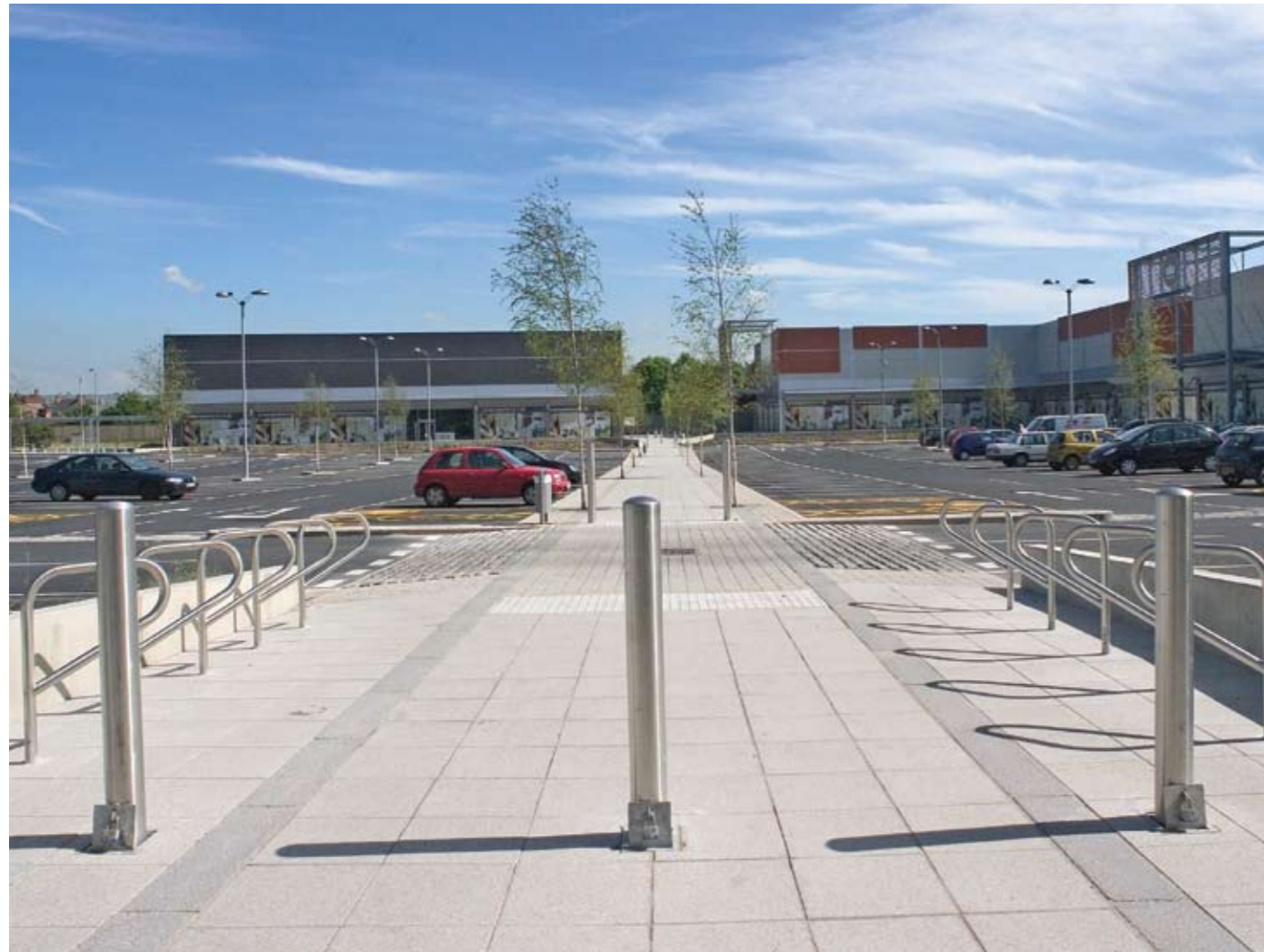
RS 001 lift out lockable bollards with Sineu Graff Diamond Point Elliptical litter bins and bespoke cycle parking on Conservation Paving, Crown Point, Denton
